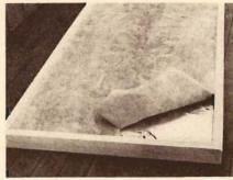
After edges are set, glue an inch of fiberglass insulation into place with butyl-rubber cement from adhesive caulking tube. Pipe grid goes on top.
