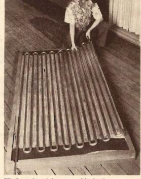
Seat the piping assembly in the beadboard box. Paint flat black, then attach glazing in plywood frame; bolts along edges hold it together.
