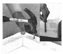
2 To form a tray for the piping, glue beadboard strips to flat beadboard panel, driving in \(^{4}\)" wood dowel to hold surfaces together firmly.
