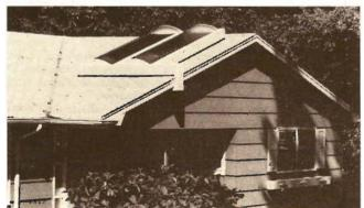
Curved acrylic collector covers look nicer and make snow readily slide off. Absorber plate is aluminum; maker says distilled water/antifreeze solution will not corrode. Heat ex-
